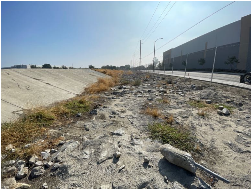
Photo 6. View facing east of rip-rap spillway along the southern project boundary.
